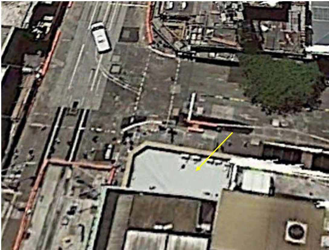
Figure 6-28 – Aerial view of Former Skinners Family Hotel, 2018 showing roof form modified since 1943 indicated by an arrow. Source: GoogleEarthPro, December 2018.
